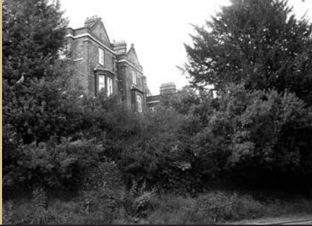
Rear of Boarding houses on Grove hill
