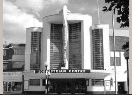
Former Ace Cinema Alexandra Avenue
