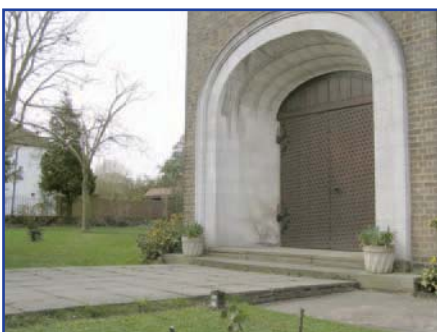
St Anselms Church before access improvement work
