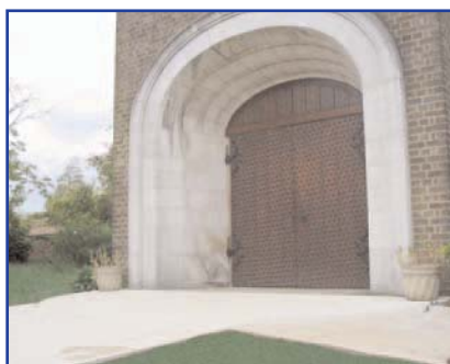
St Anselms Church after access improvement work
