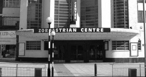
Stagger bond paving outside cinema
