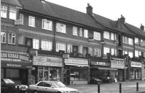
Simple traditional shopfront with narrow fascia
