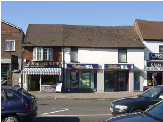
81-83 High Street (locally listed buildings)
